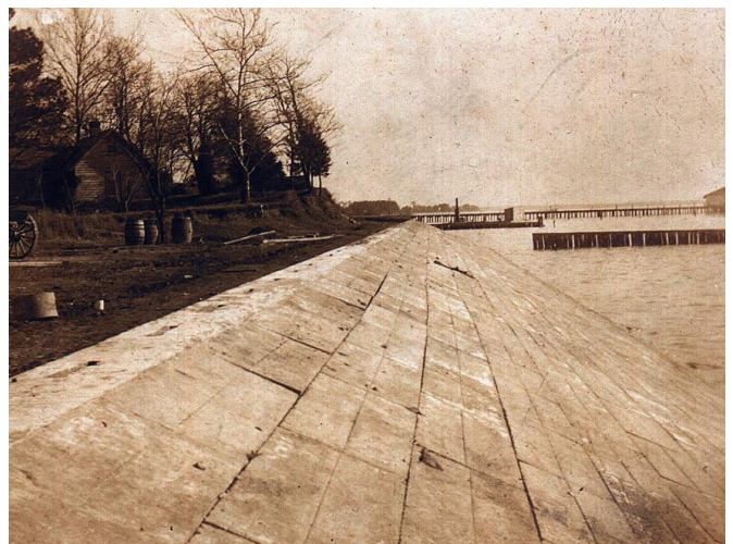
Top: The APVA's first attempt at erosion control in the 1890s. Bottom: The 1906 seawall designed by Samuel H. Yonge.
