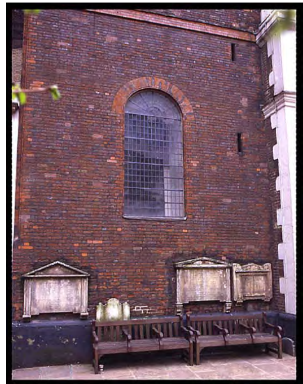
St. Peter upon Cornhill (1677-84), London. Designed by Sir Christopher Wren. Note the use of rubbed work in the stringcourse, surrounding the window, and at the corner. Heavy quoins, as used at places such as the Black Horse Inn, have been eliminated, but Wren has still had the corner sculpted with carved brick. Photograph by Willie Graham, 2001.
