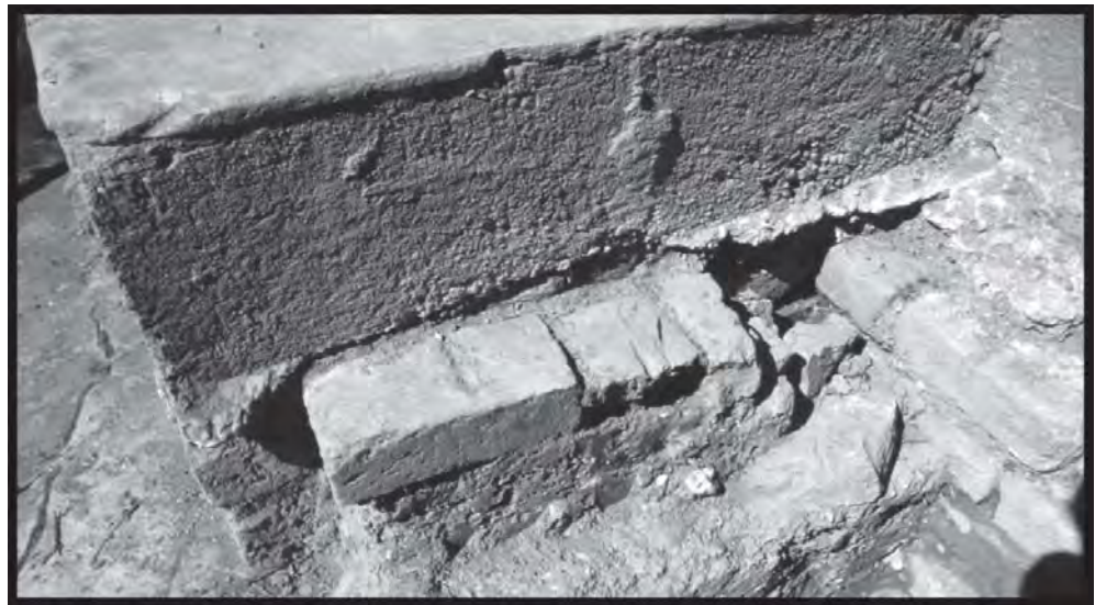
Detail of rubbed hearth brick, east chimney, House 4. Photograph by Willie Graham, 2001.
