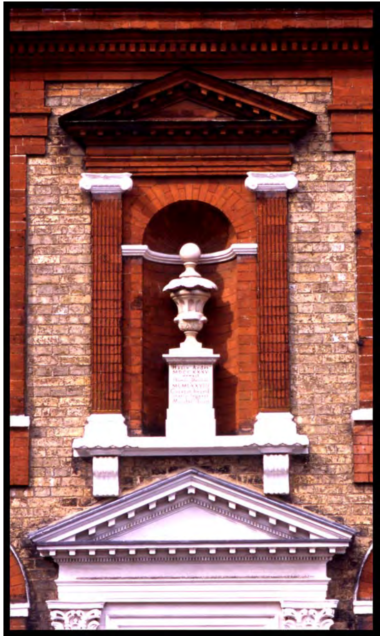
Thomas Sherman House (1735), Dedham, Suffolk, England. Carved gauged-and-rubbed work is used in this eighteenth-century house to contrast with its yellow wall brick. Photograph by Willie Graham, 2001.
