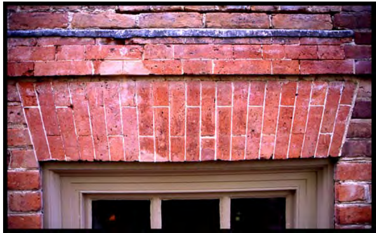
Although wide openings for casements were initially laid out at the College of William and Mary when work began in 1695, workmen were immediately directed to switch the proportions for installation of sash windows. Above cellar level, gauged-and-rubbed jack arches spanned the openings, here seen tucked beneath the stringcourse with its lead capping. Photograph by Willie Graham, 2001.
