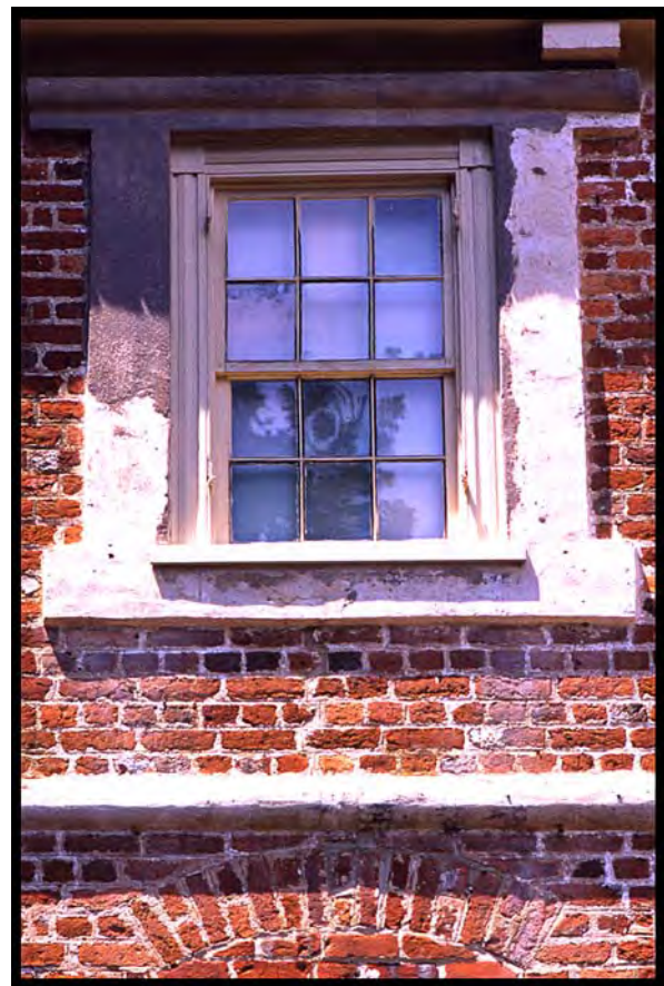
Above: detail, front façade of Ravensmere (1694), Beccles, Suffolk, England. This finely crafted stringcourse has a molded top and bottom course, is made of precisely gauged-and-rubbed brick, and stops short of the corners. Note also the use of carefully chosen orange stretchers and contrasting black, glazed headers arranged in a Flemish bond pattern for the wall. Photograph by Willie Graham, 2001. Below: Molded and stuccoed stringcourse at Bacon's Castle in Virginia. Photograph by Willie Graham, 2001.
