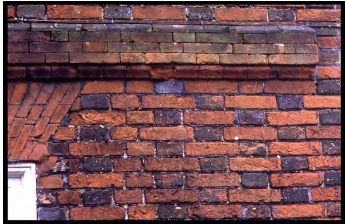
Above: detail, front façade of Ravensmere (1694), Beccles, Suffolk, England. This finely crafted stringcourse has a molded top and bottom course, is made of precisely gauged-and-rubbed brick, and stops short of the corners. Note also the use of carefully chosen orange stretchers and contrasting black, glazed headers arranged in a Flemish bond pattern for the wall. Photograph by Willie Graham, 2001. Below: Molded and stuccoed stringcourse at Bacon's Castle in Virginia. Photograph by Willie Graham, 2001.
