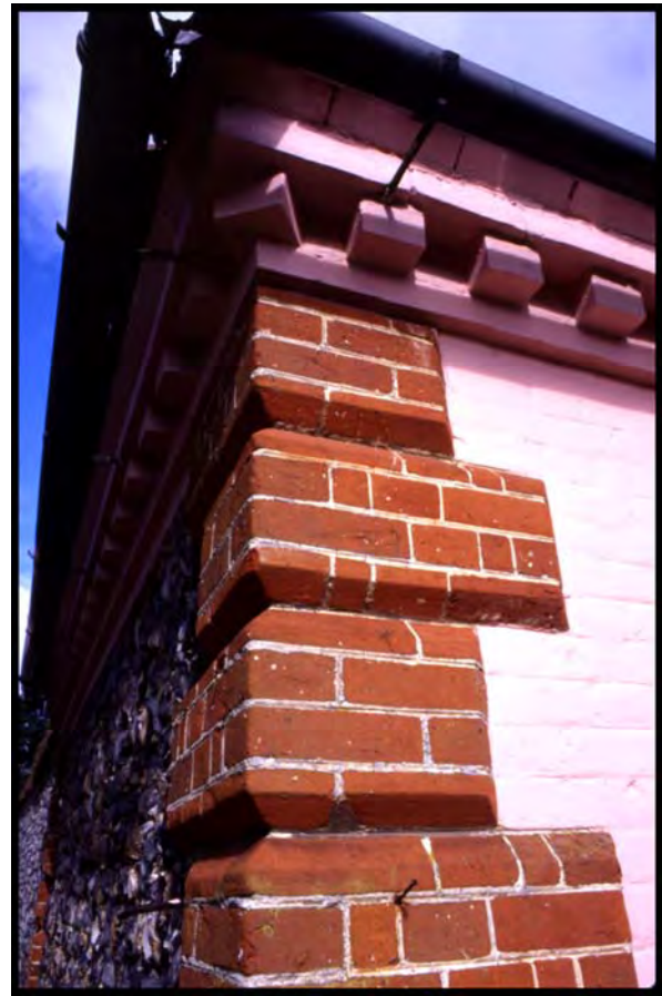
Brick modillion cornice and carved gauged-and-rubbed quoins, Ampton Almshouse (1693), Suffolk, England. Photograph by Willie Graham, 2001.
