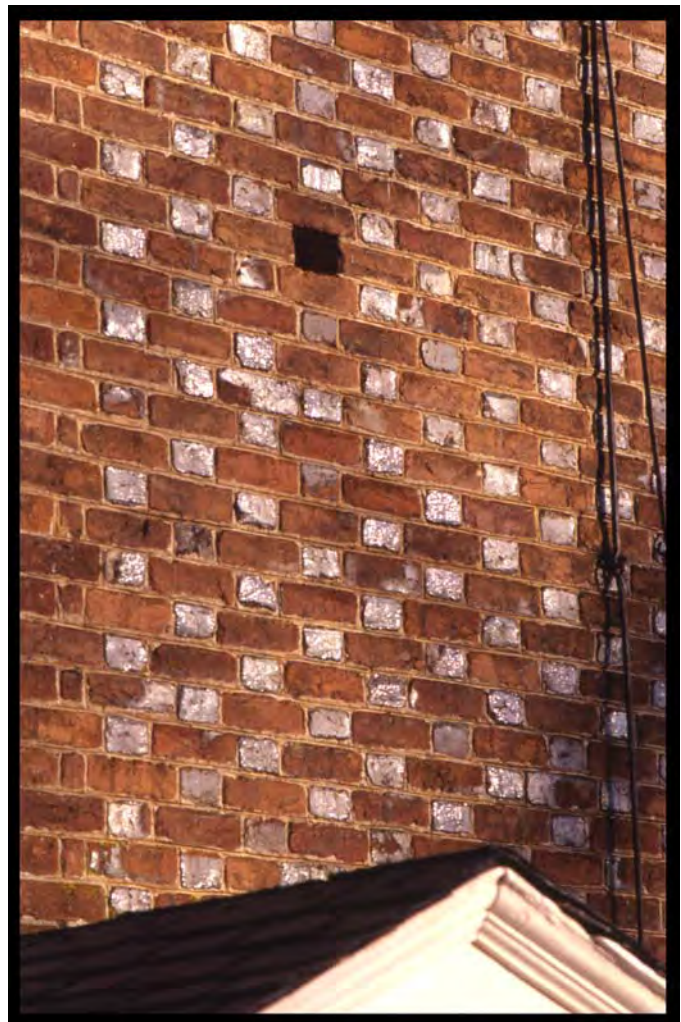
All-glazed header Flemish bond brick gable at Tuckahoe, Goochland County, Virginia, dating to about mid century. Photograph by Willie Graham, 1998.
