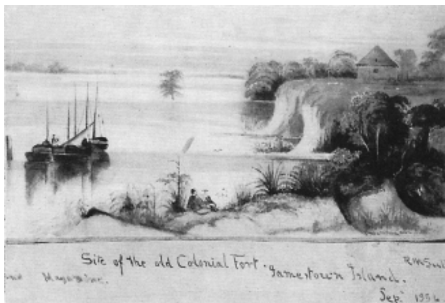
Figures 3, 4, 5. Engravings and paintings of the churchyard at Jamestown before construction of the Civil War earthwork all suggesting that the shoreline was much higher before that massive earth-moving construction took place.
